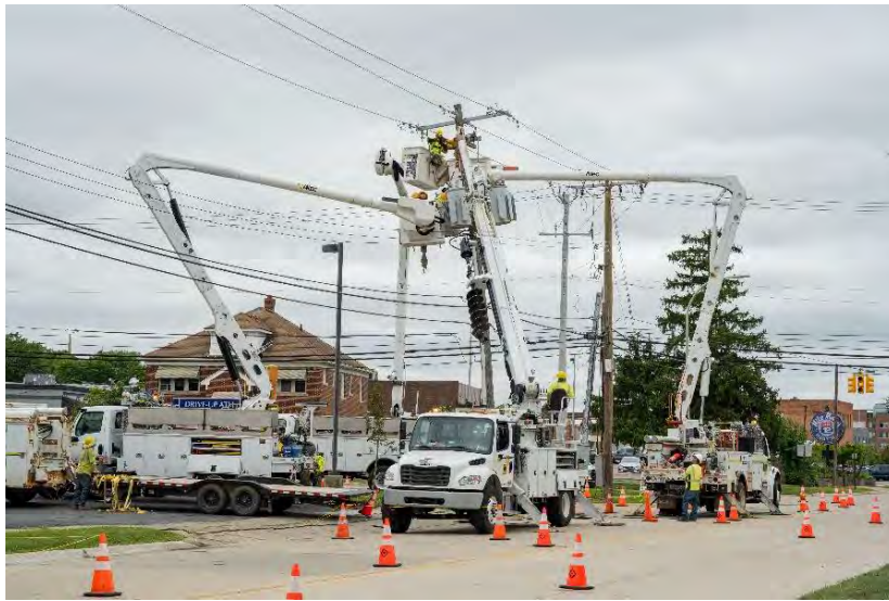
Conversion work in Wayne
