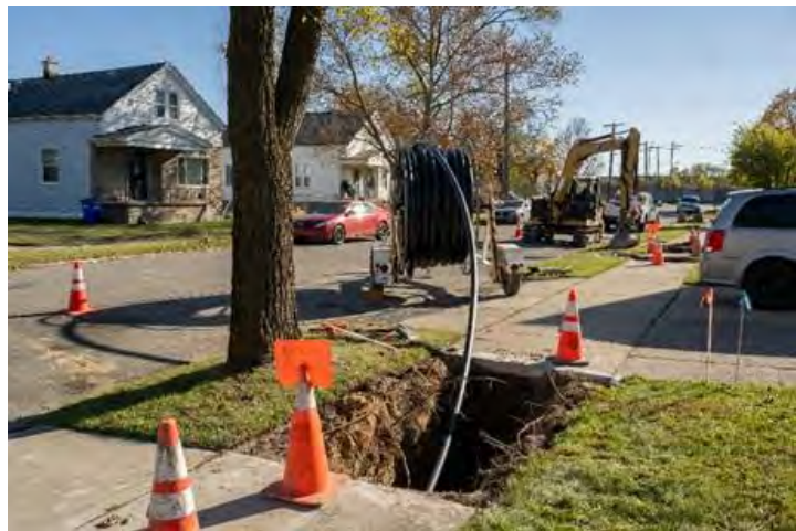
Undergrounding work on Buffalo Charles project
