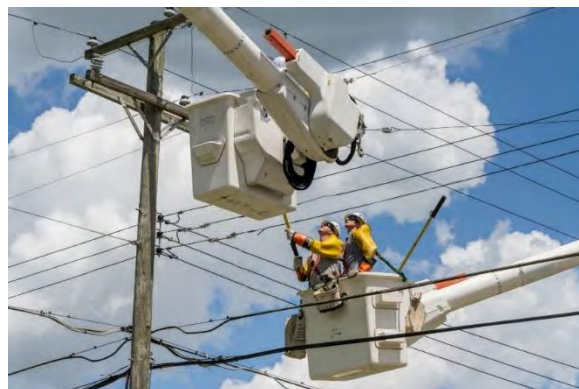
Linemen restoring power
