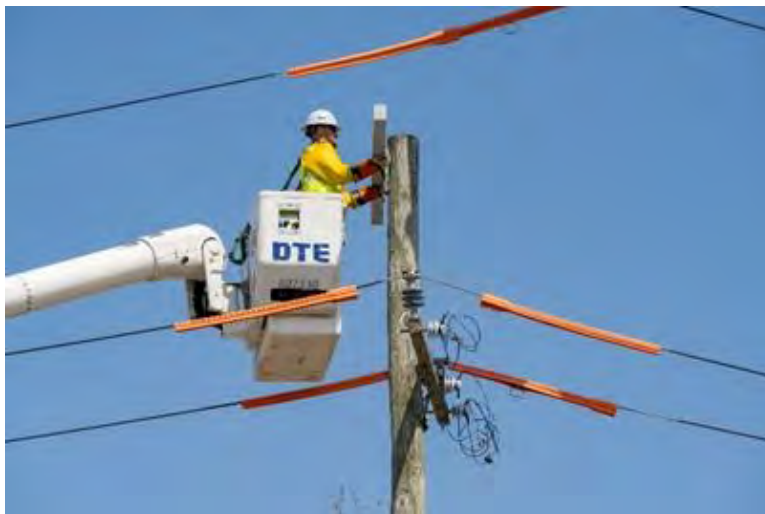
Lineman installing fiberglass crossarm
