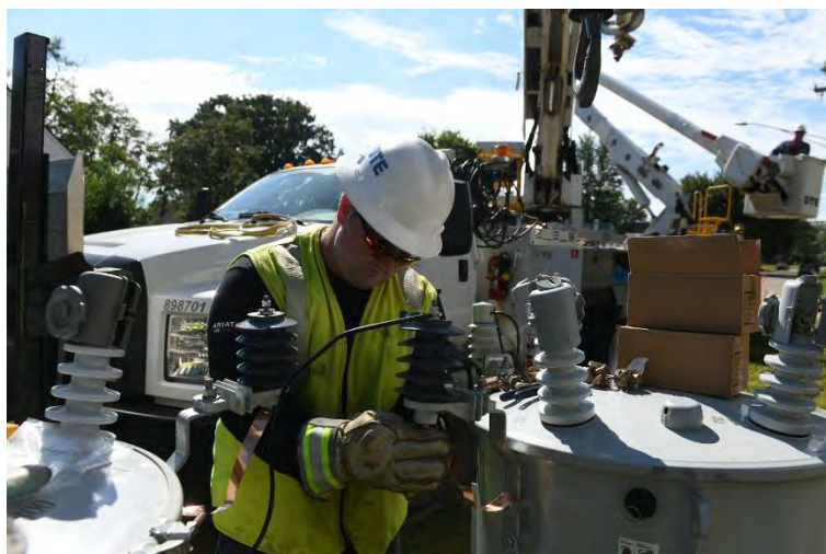
Lineman works to install a new set of transformers
